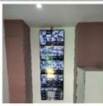
Cabling Works, CCTV and Monitors Installation
