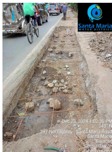
Brgy. Guyong, National Road from Gravador St. to Celestino St. 150mm Diameter Mainline Pipe Replacement Project
